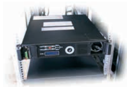
Carry out manual bypass operation on faulty unit selecting S1 or S2
